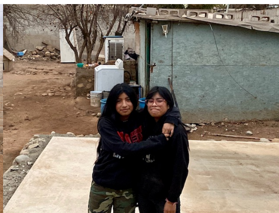
S&K standing on the new slab
